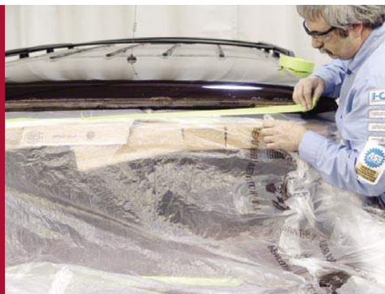
Figure 3 - The vehicle interior must be protected from the repair process.
