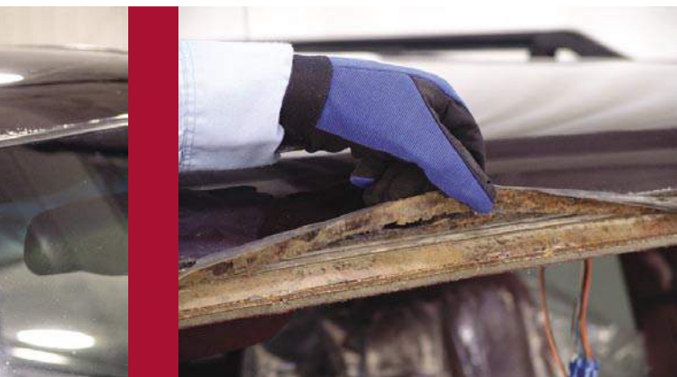
Figure 2 - This vehicle has extensive corrosion damage beneath the urethane that may have inhibited the safety features of the windshield.
