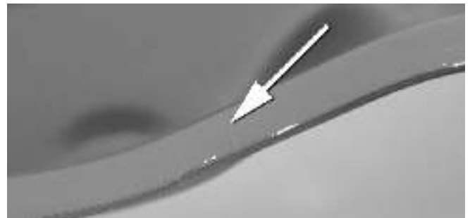
Figure 5 - This joint shows no difference in thickness between the steels.
