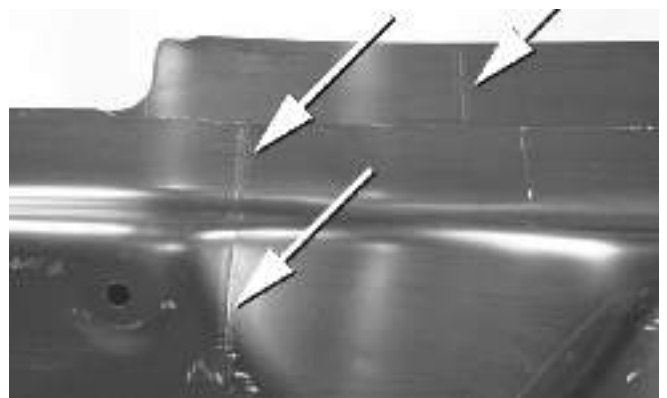
Figure 6 - Laser welds on this lower rail or side member show offset joints between the inner and outer halves.
