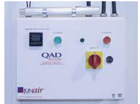
Figure 5 - The control unit is mounted on the outside of the spraybooth and is used to turn on the system.
