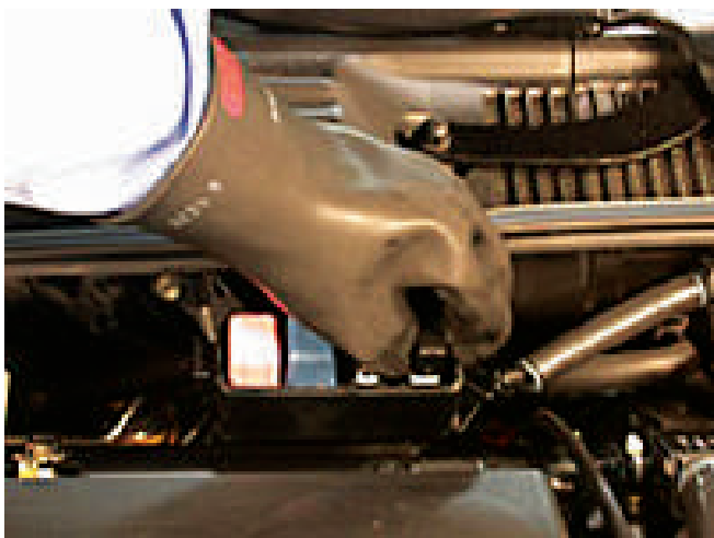
Figure 2-Removing this relay under the hood will also disable the high voltage system on the Toyota Prius.
